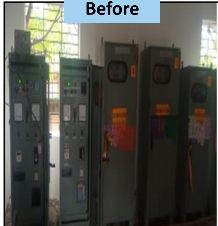
Replacement of old non-communicable CR panels with new SCADA compatible panels for remote monitoring and operations by PSSC, at central level.
