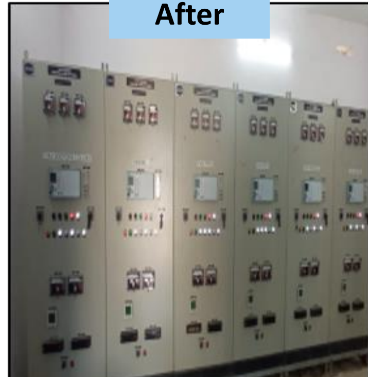
Replacement of old non-communicable CR panels with new SCADA compatible panels for remote monitoring and operations by PSSC, at central level.
